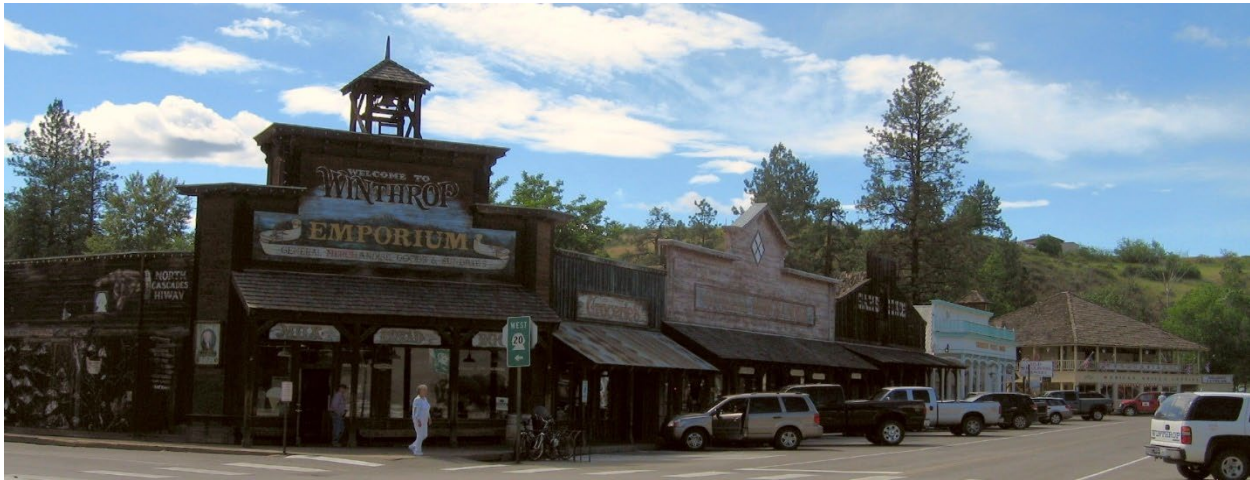
Figure 3.c.14. Winthrop is the main choke point for the upper Methow Valley for transportation, services, and recreation. A fire moving from the wildland into the urban core of the town, with its heavy utilization of wood construction inspired by the late 19 th century western aesthetic, could easily travel through the area under the right conditions. (Source: Rocklynn Culp, Town of Winthrop, nd)
