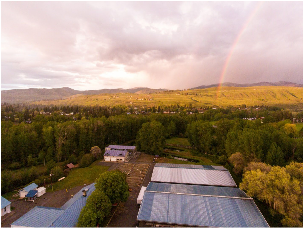
Figure 3.c.12. The narrowness of the Methow Valley leads to tight concentrations of structures within the WUI. (Source: Aaron Nepean, Cutboard Studio, 2022)
