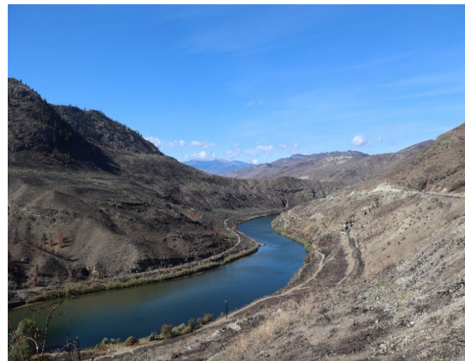
Figure 2.b.3. Post-fire impacts from the Eagle Bluff Fire in northern Okanogan County. (Source: Emmy Engle, Okanogan CD, 2023)
