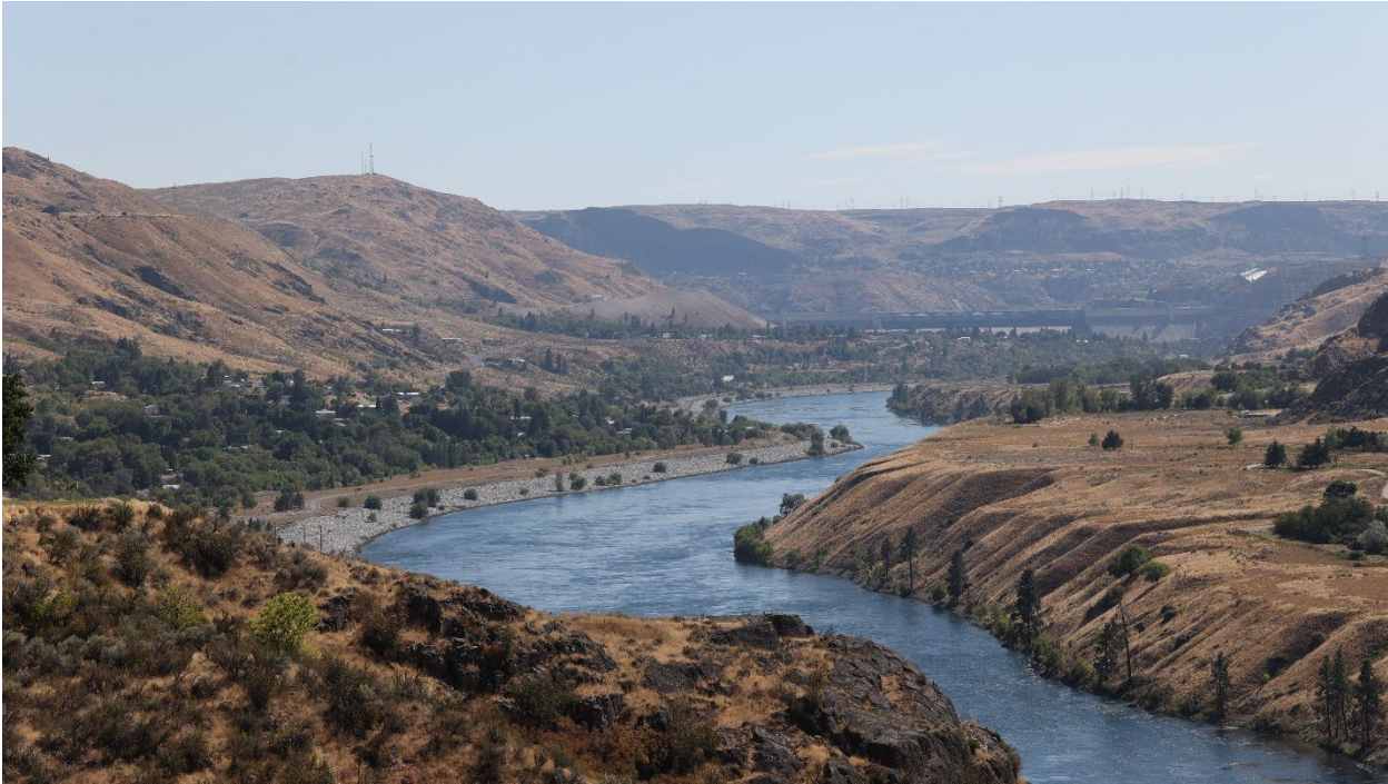
Figure 3.c.8. Overlooking Elmer City, Coulee Dam, with the Grand Coulee Dam in the background. The area is vital for the power infrastructure of the county and much of the region. (Source: Eli Loftis, Okanogan CD, 2024)
